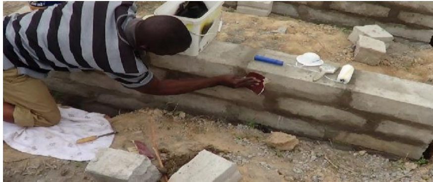
Figure 5 Surface of test wall being prepared to receive the damp proof coatings
