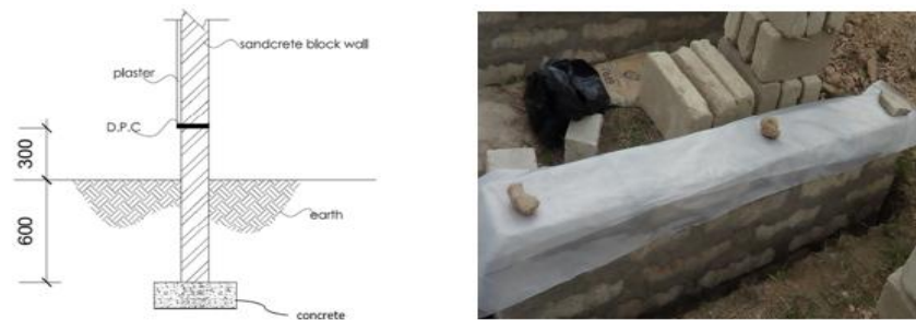
Figure 3. Diagrams showing how the polyethylene DPCs were laid
