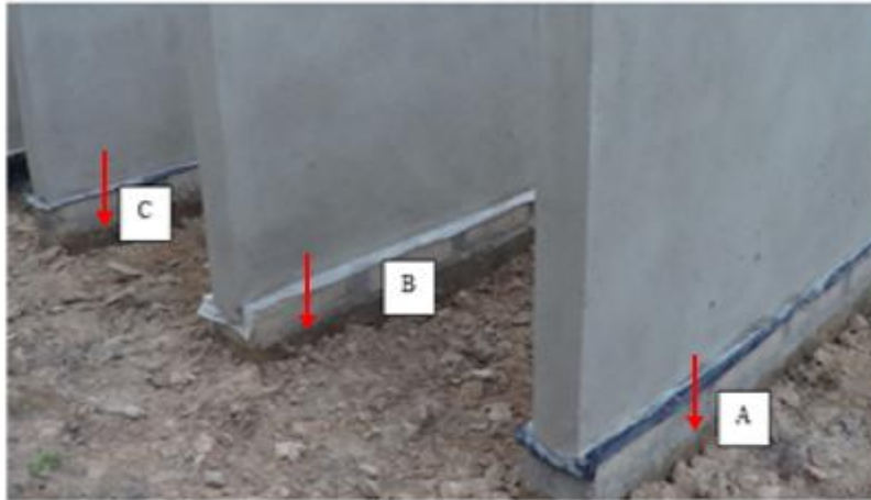
Figure 12. Water rise at the bases of the walls constructed with SBs and treated
