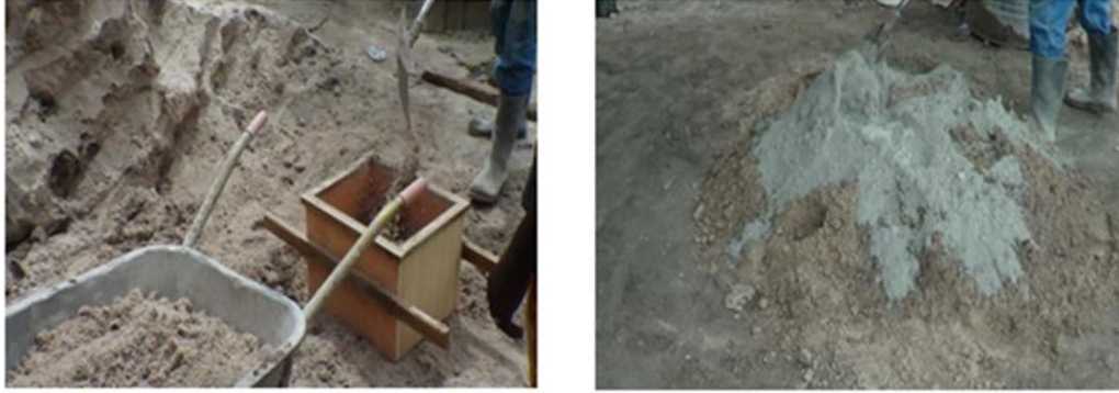
Figure 1. Volume batching of fine aggregates and cement
