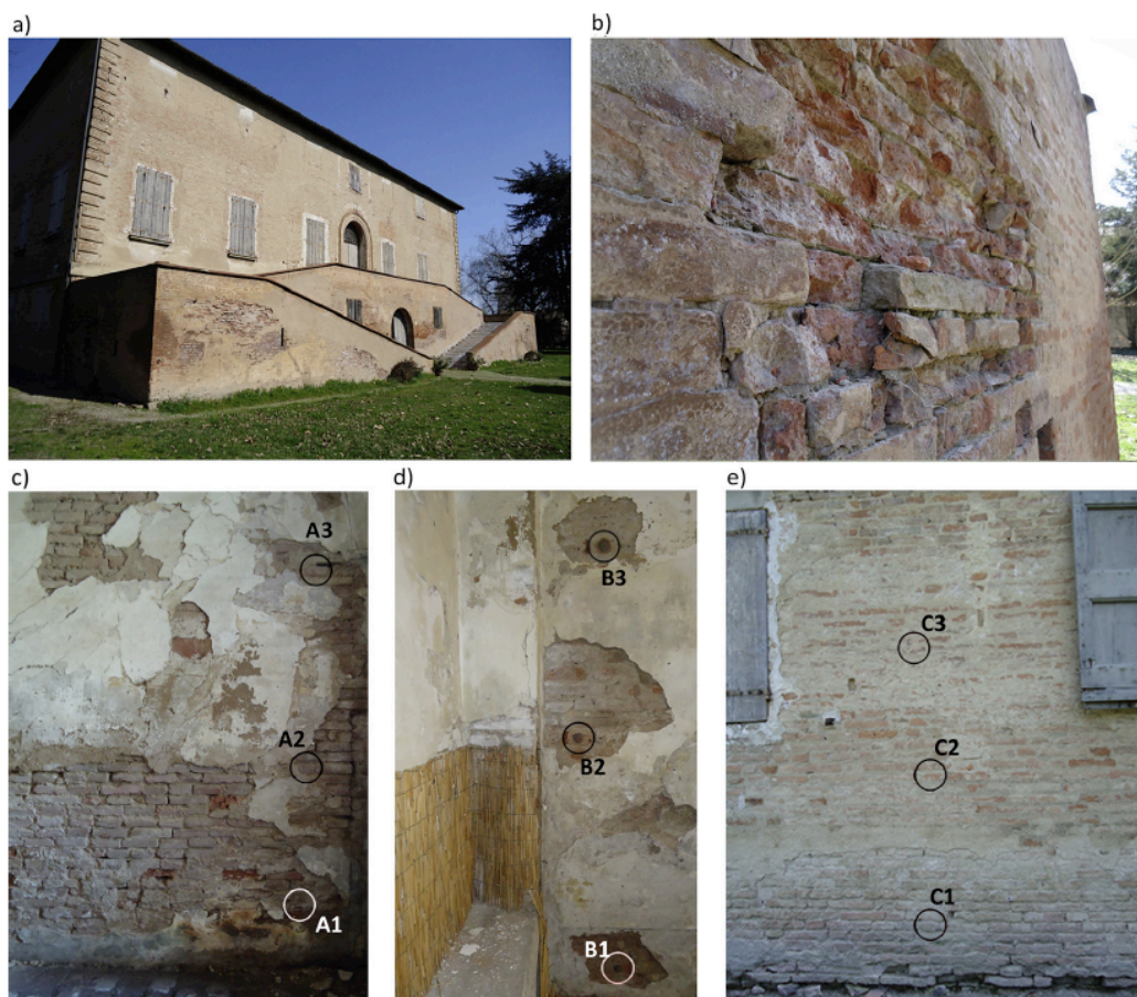
Figure 2: Isolani Palace at Minerbio: (a) North façade; (b) decay phenomenon occurring in Isolani Palace due to rising moisture and salts near zone C; (c) zone A; (d) zone B; (e) zone C.
